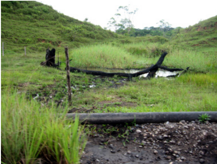
A burned tree and a pool of sludge show where the FARC guerrillas recently bombed the local oil pipeline.
